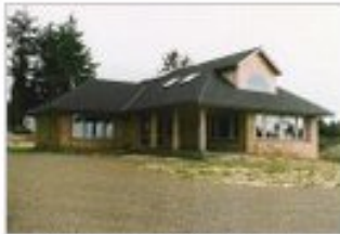
Tillamook County Library Buildings (15)
